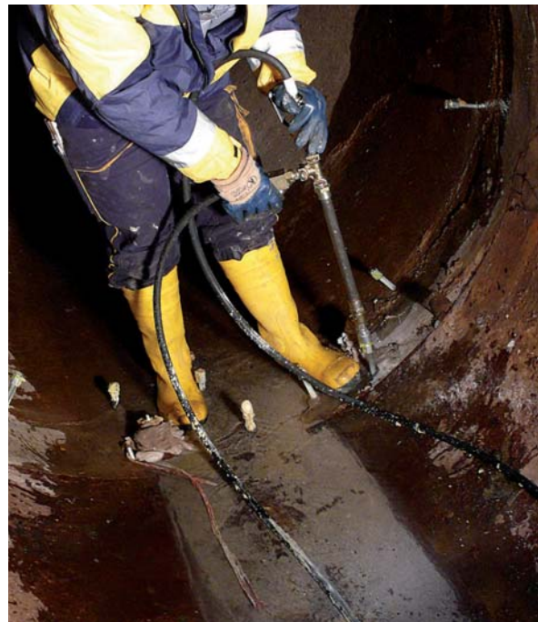
Sealing a coupling in the walkable tunnel
