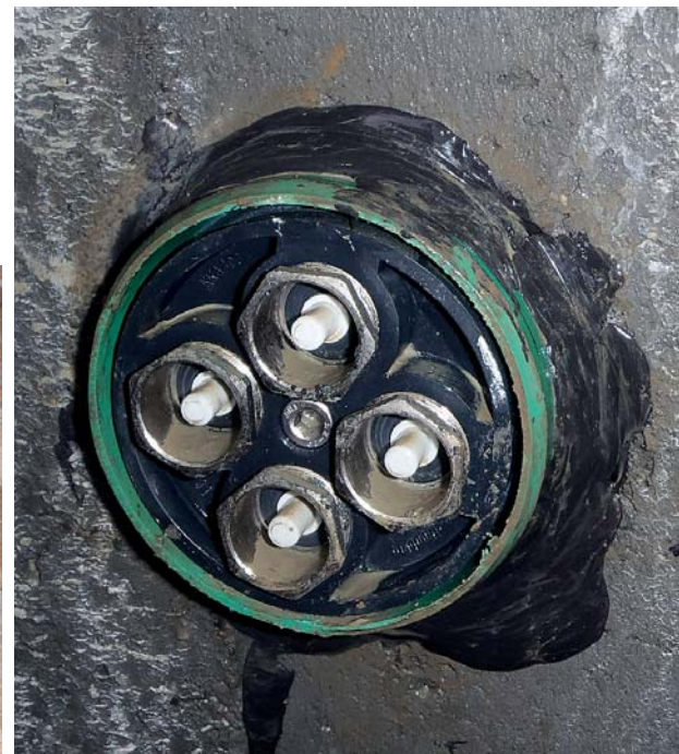
Integration of pipe into the shaft >
