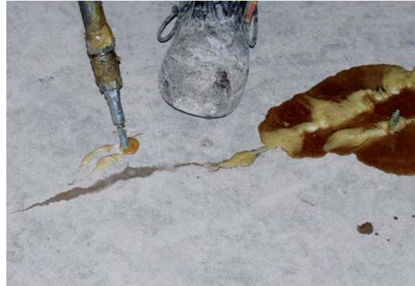
Crack injection
