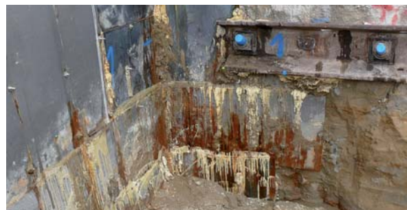
Plating and sealing a high-pressure soil cementation
