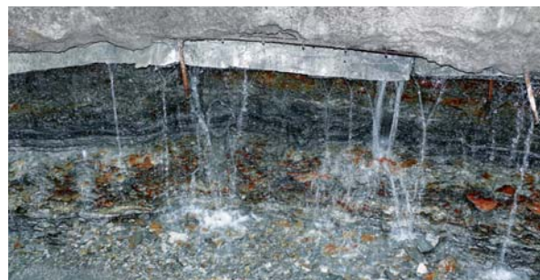
Leaking shotcrete shell during the drilling of a shaft
