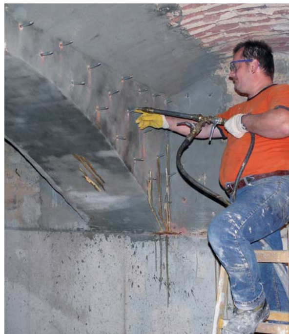
Improving the load capacity of an arch
