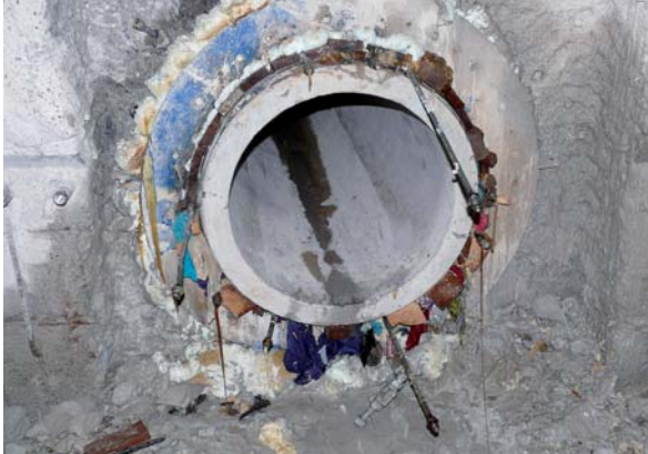
Ring gap after injection
