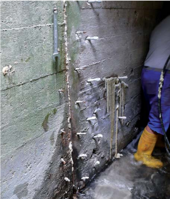
Joint after sealing
