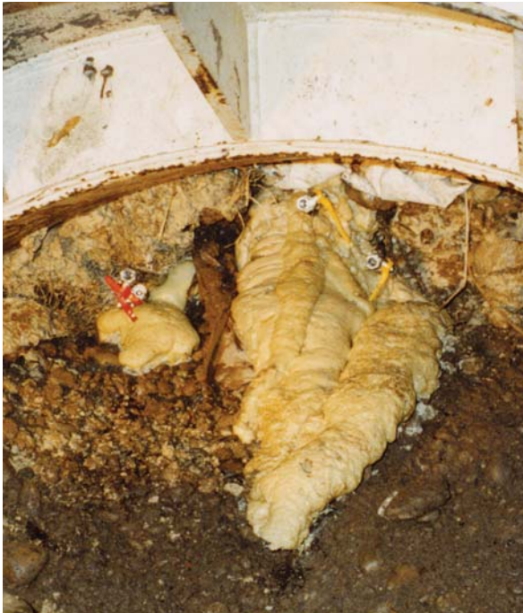
Advance consolidation of loose gravels
