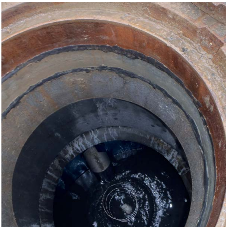
Sealing of the shaft ring joints
