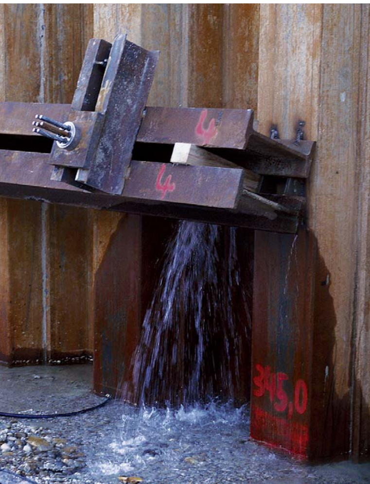
Leaking shotcrete shell during the drilling of a shaft
